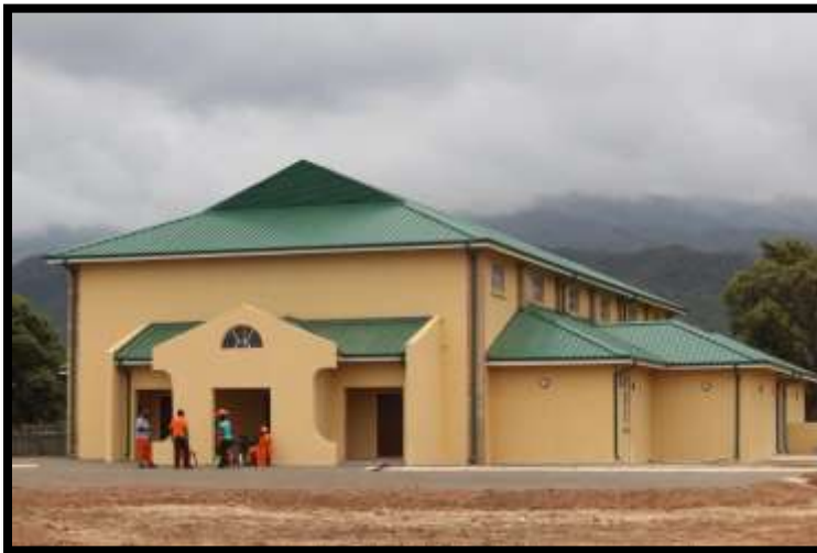
Moshate Community Hall
